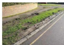
Parking causing damage to the verge
